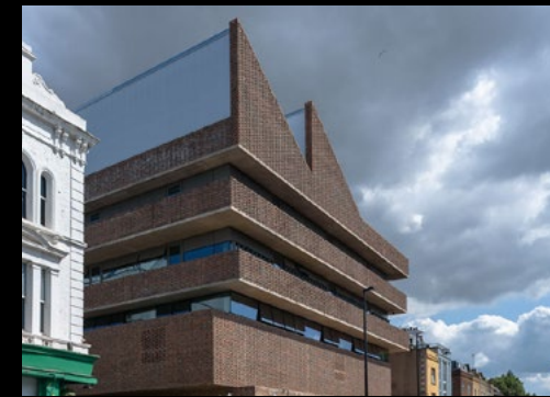
New Battersea Campus
